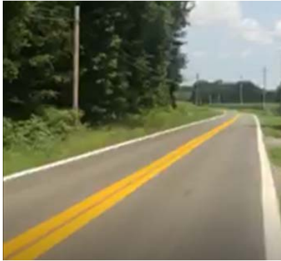
Widened edge and center lines
