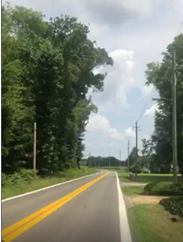
White and yellow striping widened from 5' to 10"
